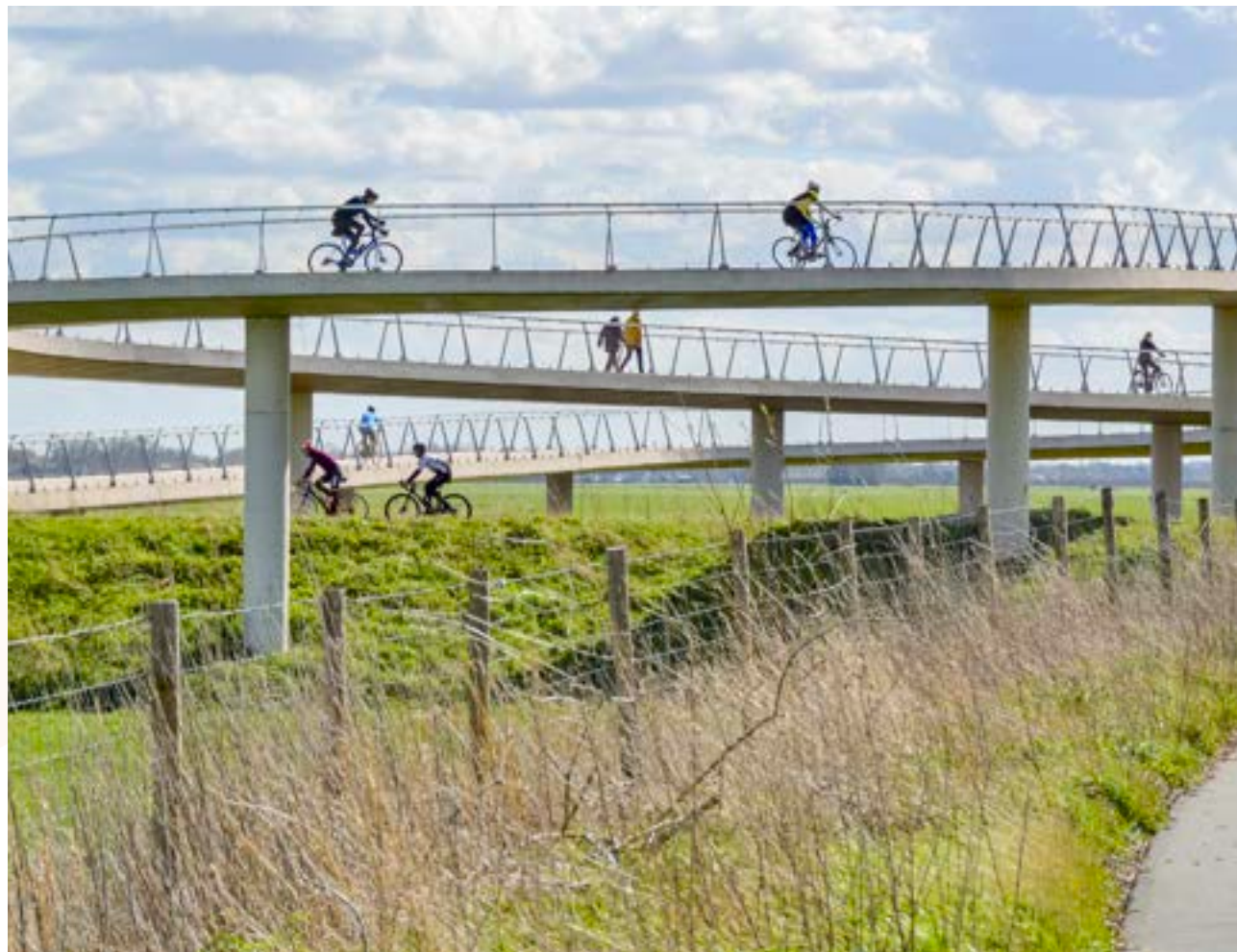
Bicycle bridge in Nigtevecht, Netherlands Source: Dutch Cycling Embassy
